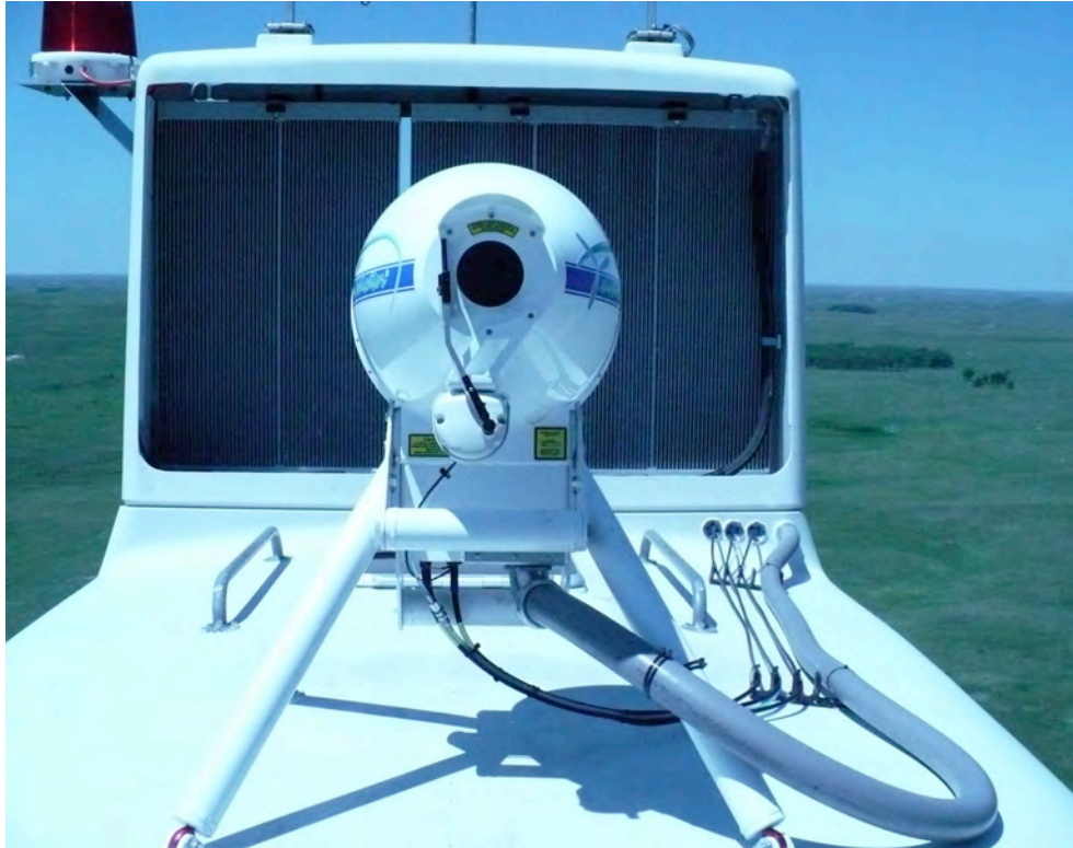
Figure 1 Vindicator ® LWS Installed on T22
